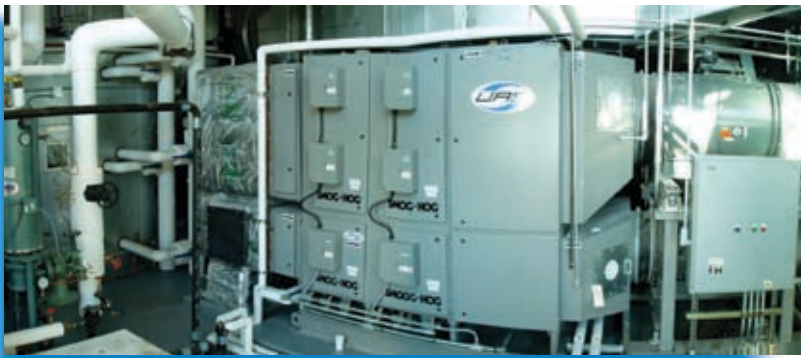
Hearst Tower installation
