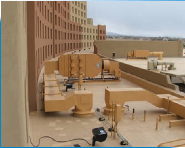
Sandia Resort & Casino installation
